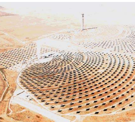
Abengoa - New CSP solar plants near Seville (Spain)
