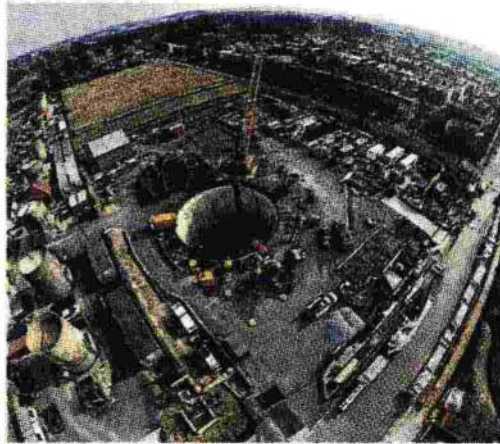
Qui sopra, il First Street Tunnel project a Washing- ton
